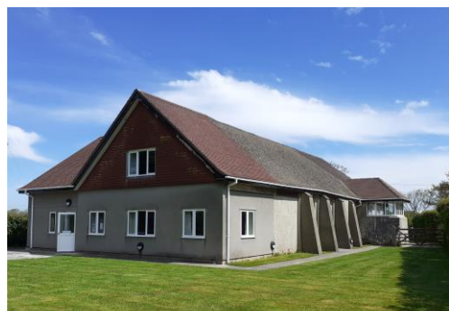
Main Hall from rear showing perimeter path, and rear entrance.
